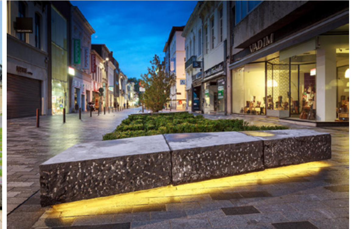
Lighting strip feature at the bottom of the stone element, split face finish at front.
