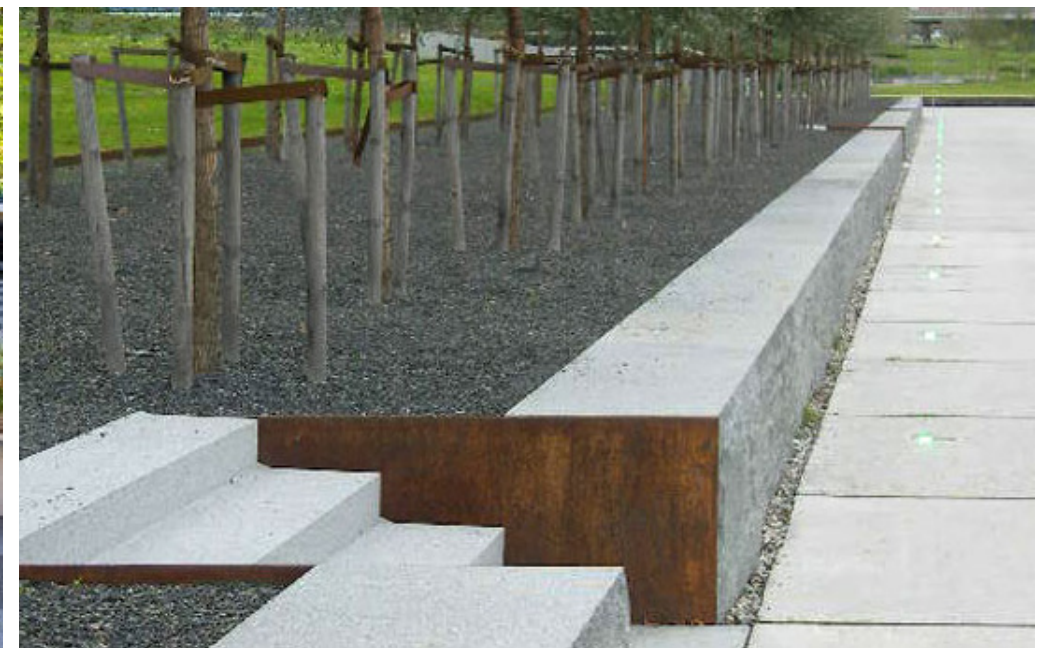
Reference for Crab apple tree orchard planters: stone edge only from one side, all other 3 sides of the planter are corten steel.
